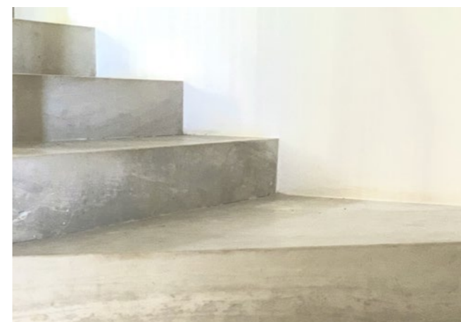
Scala levigata | Honed finish stairs
